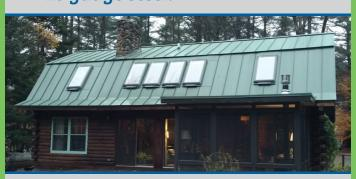
2. Standing seam metal roofing has very few exposed fasteners.
